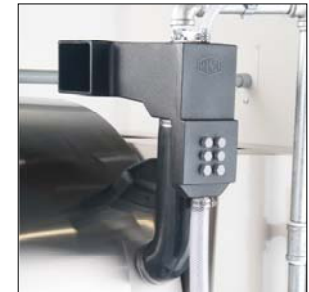
Safe chemical injection
