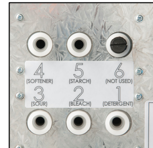
Safe chemical injection
