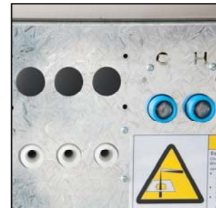
Safe chemical injection
