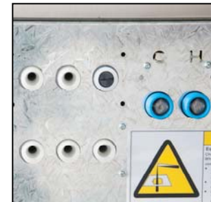
Safe chemical injection
